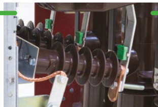
TH110 sensor mounted on cable termination
